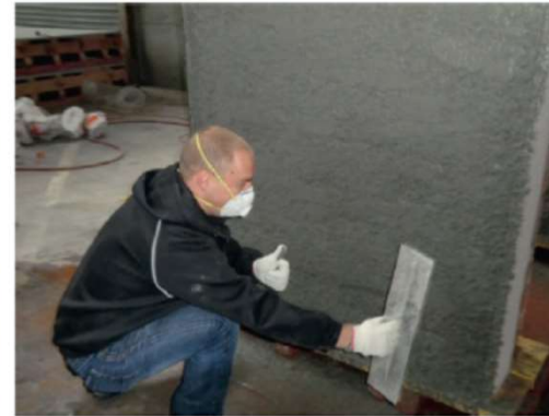
(c) Trowelling sprayed ECC flat prior to the spraying of successive layers
