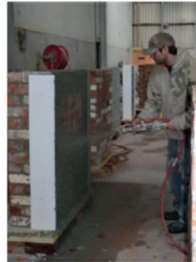
(b) Spraying of ECC shotcrete onto walette
