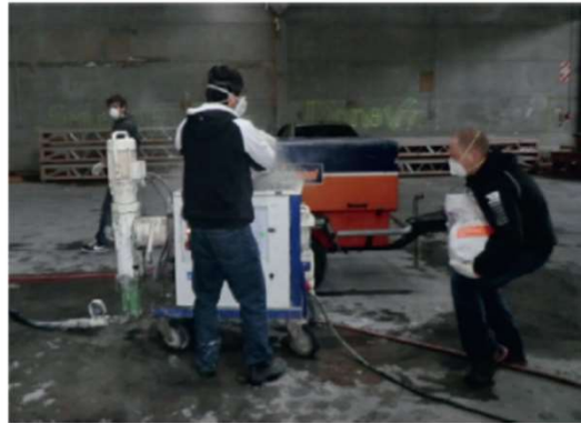
(a) Adding prebagged ECC into mixer
